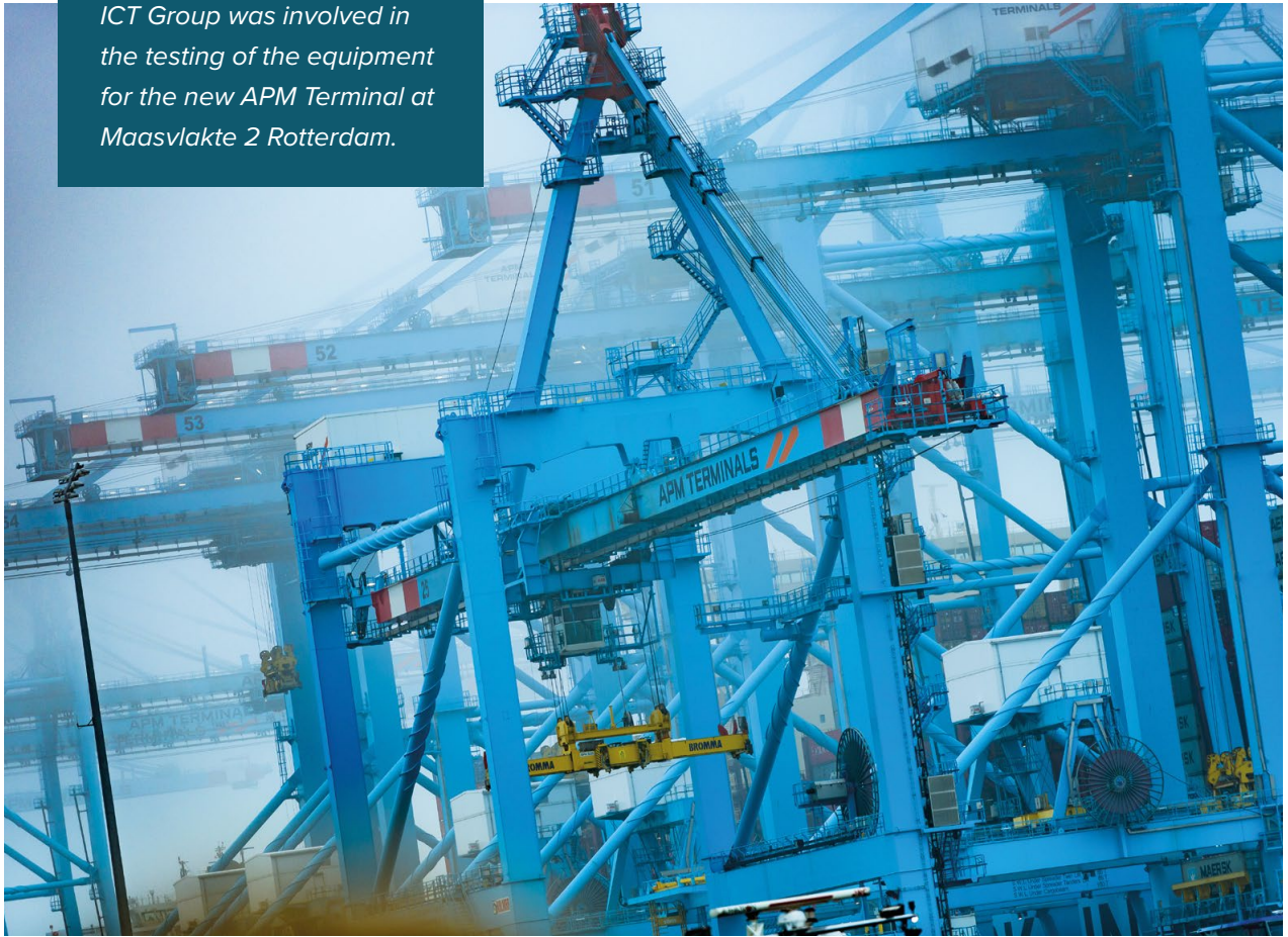
QC - Quay Cranes
